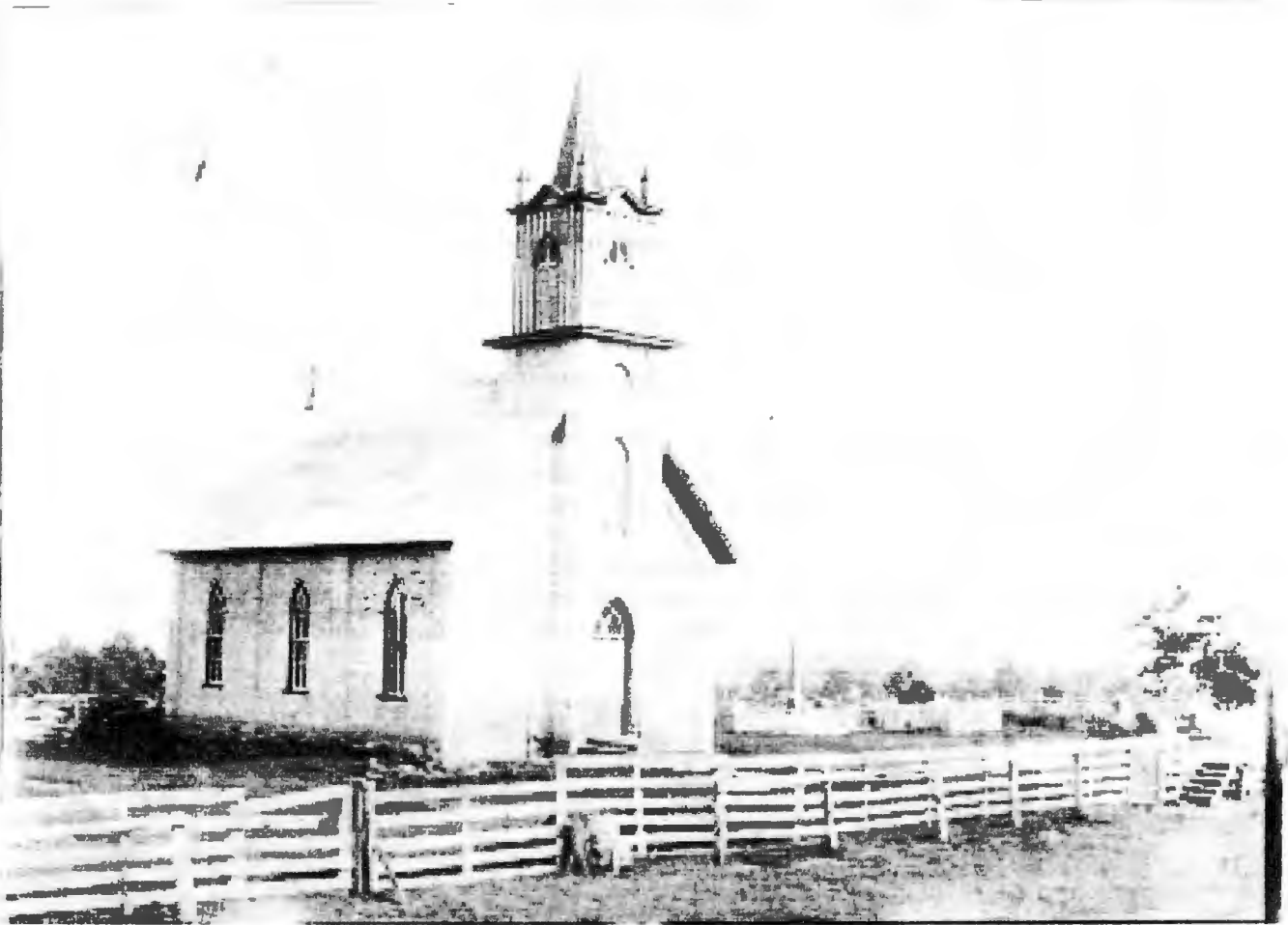
The Westfield German Methodist Church , circa 1880. Church records show that the fence was in constant need of repair
