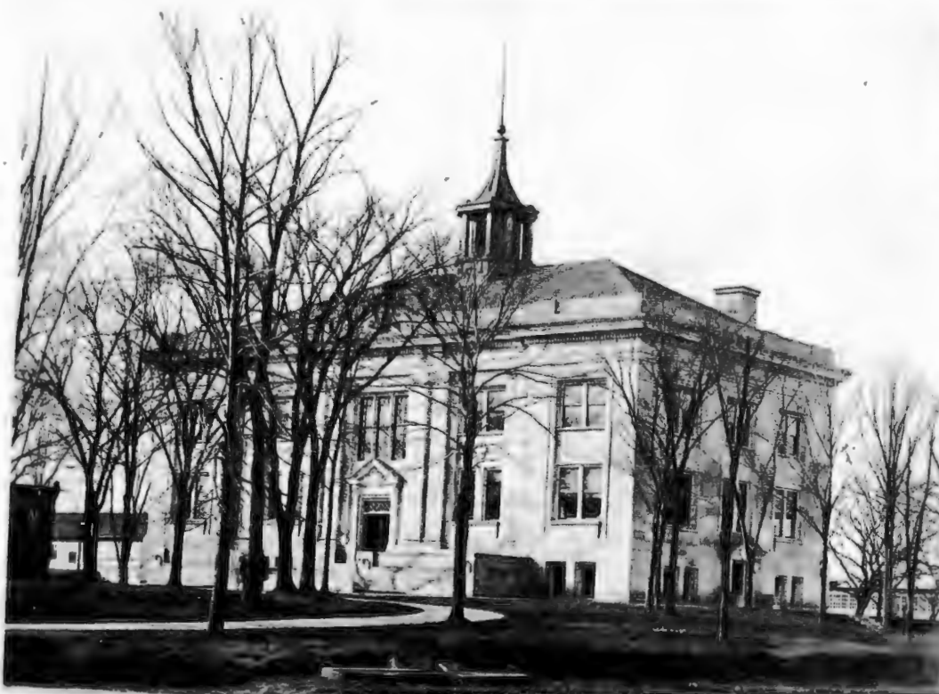
The 1905 Court house before additions to the west
