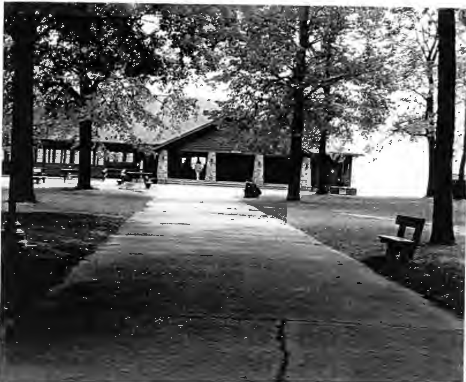
Though the road bypasses it now, the original cement of the Warner Memorial Road can be seen directly in front of the Chateau at Devils Lake
