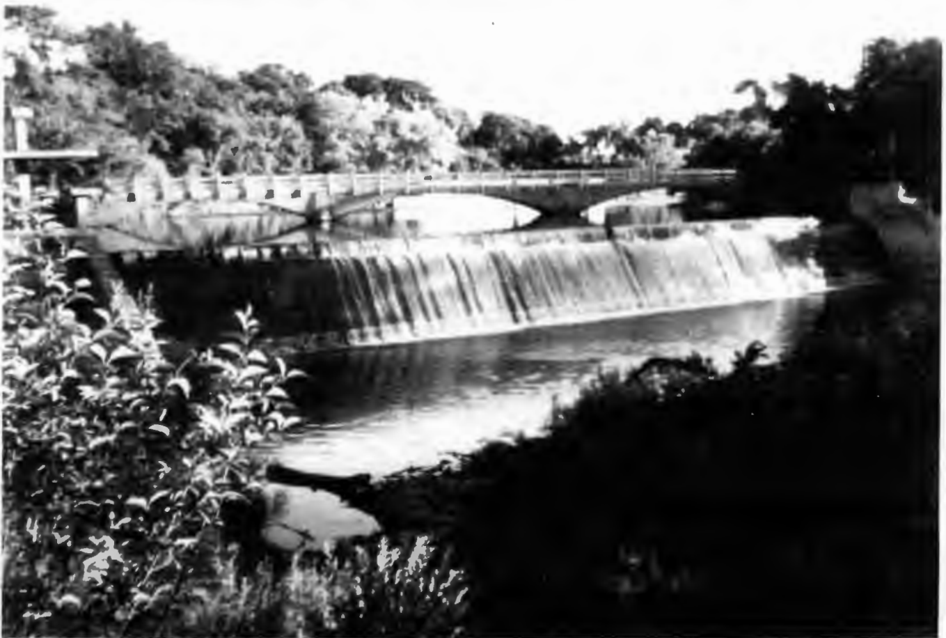
The Island Woolen Mill Bridge and Dam
