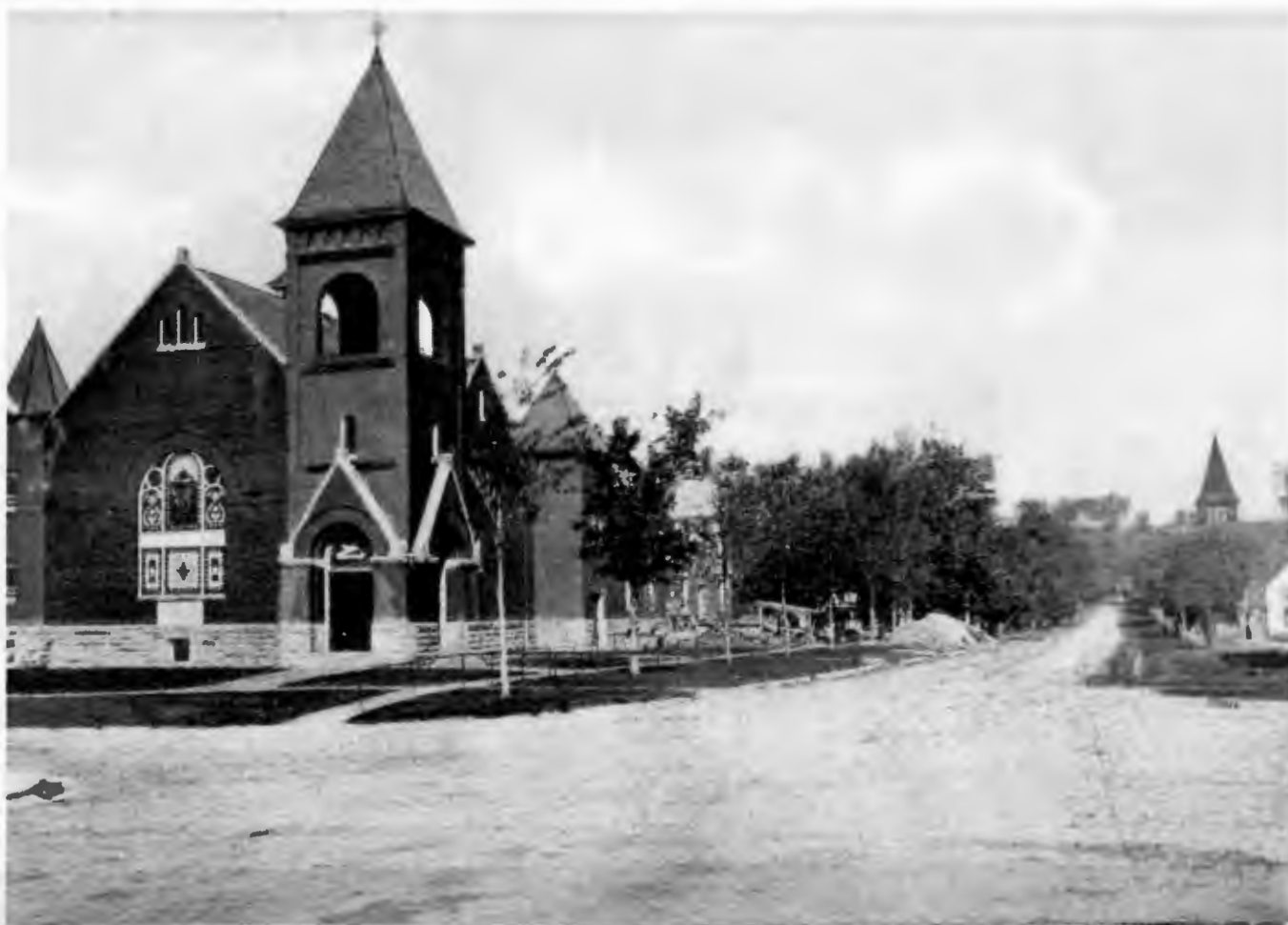
1904-5 The "new" Methodist Church. Work continues on Al Ringling mansion in the distance
