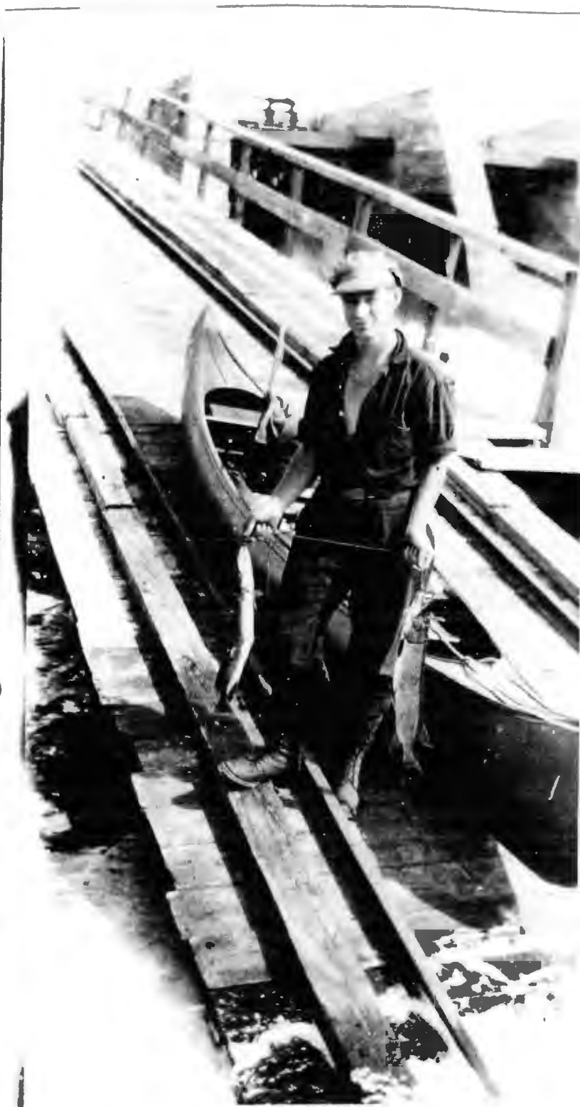
Clausen Stekl at the dam at Grandfather Falls
