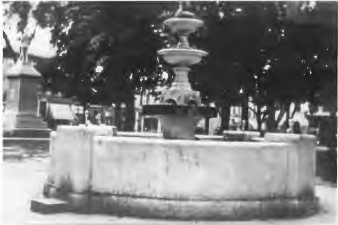
The Courthouse Drinking Fountain was popular during Prohibition
