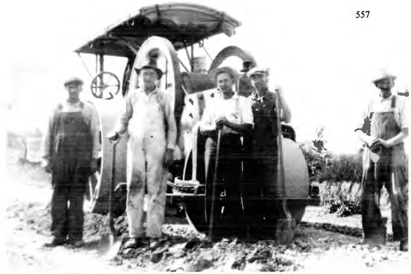
U.S. 12 was paved using both steam rollers and men with shovels.
