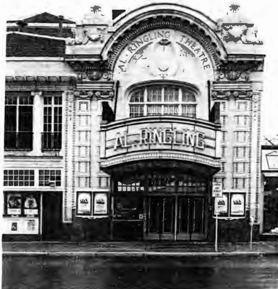
In 1937, Rapp & Rapp was commissioned to encase the original marquee within the current model, with the Al. Ringling name in glowing lights. (Douglas C. Green, Historic American Building Survey.)
