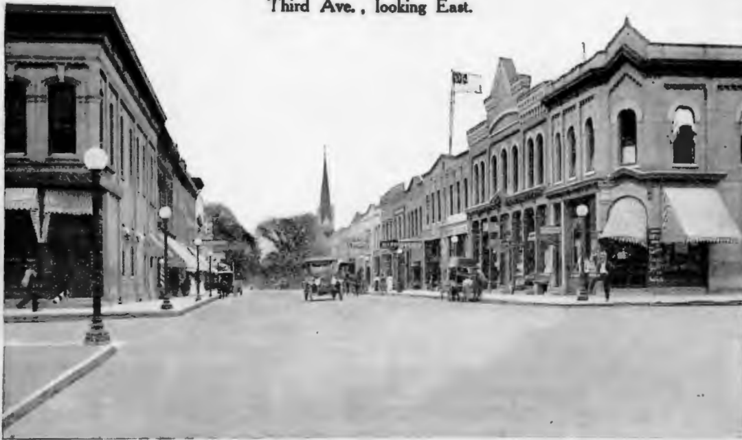
Third Ave. , looking East.
