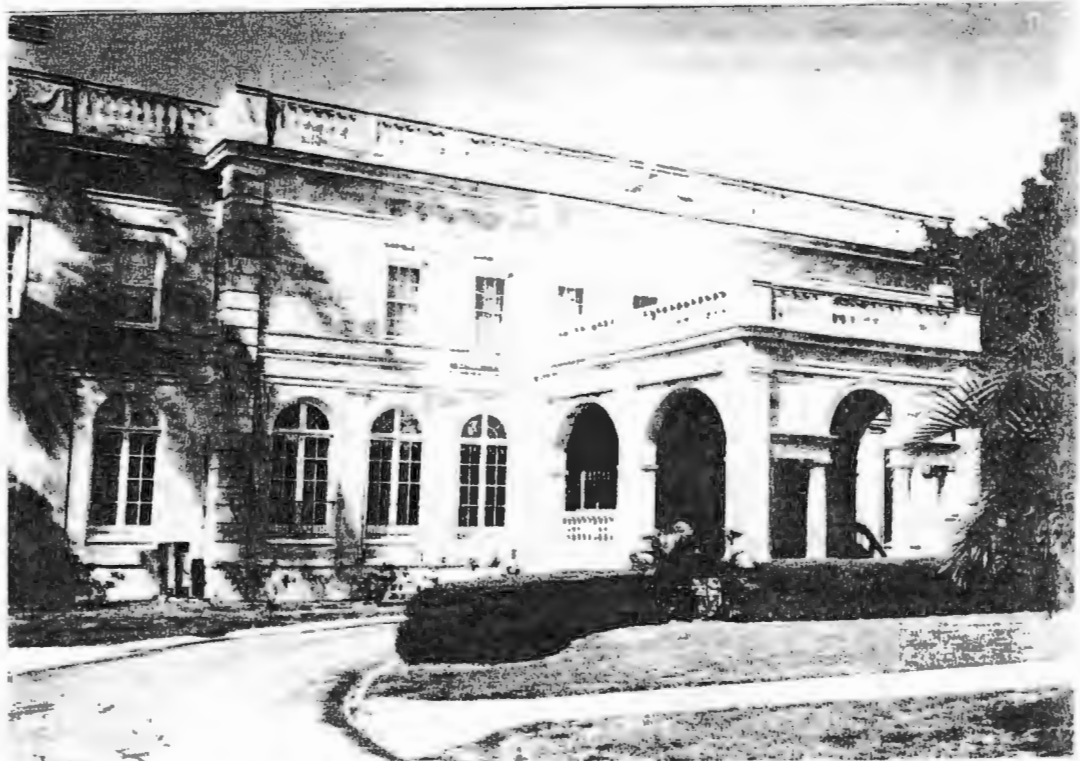
Entrance with porte cochere
