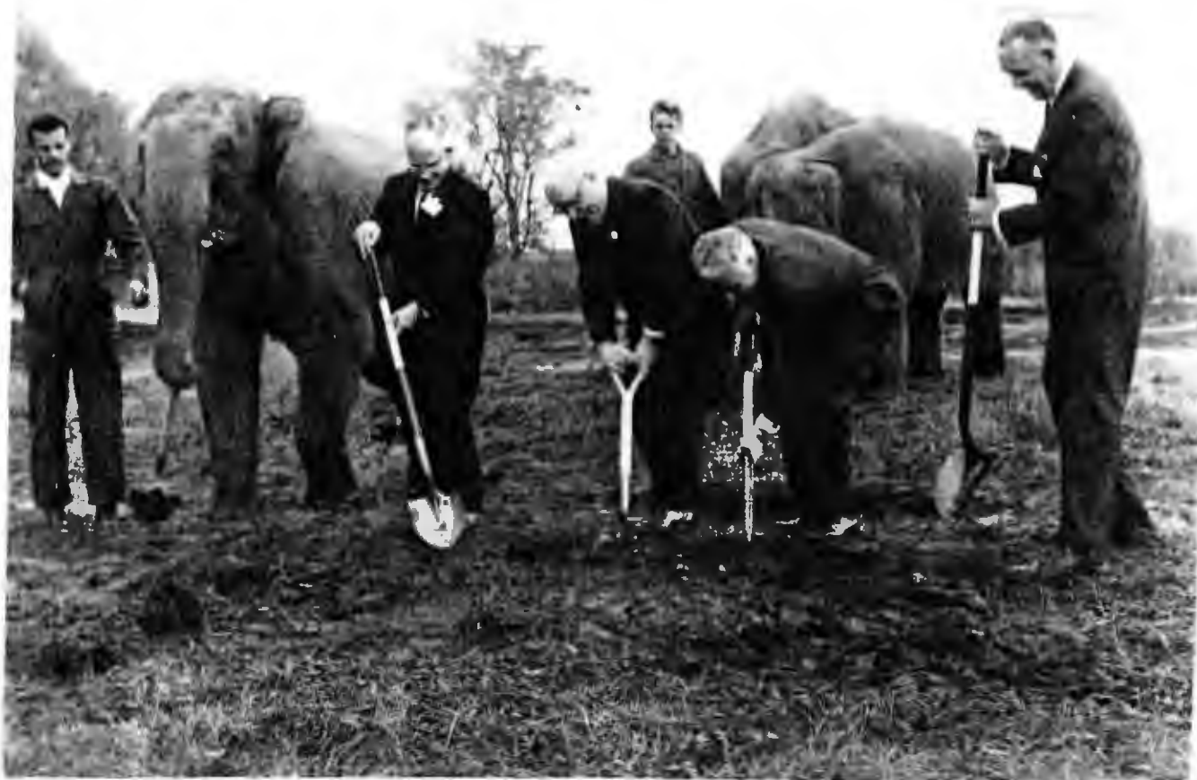
Elephants assisted at the ground-breaking for Eagle Signal. From the left: elephant trainer John Herriot, plant manager Chester Corson, Carl Anderson of E.W.Bliss, Gov. Warren Knowles, and Mayor Bill Hommel.
