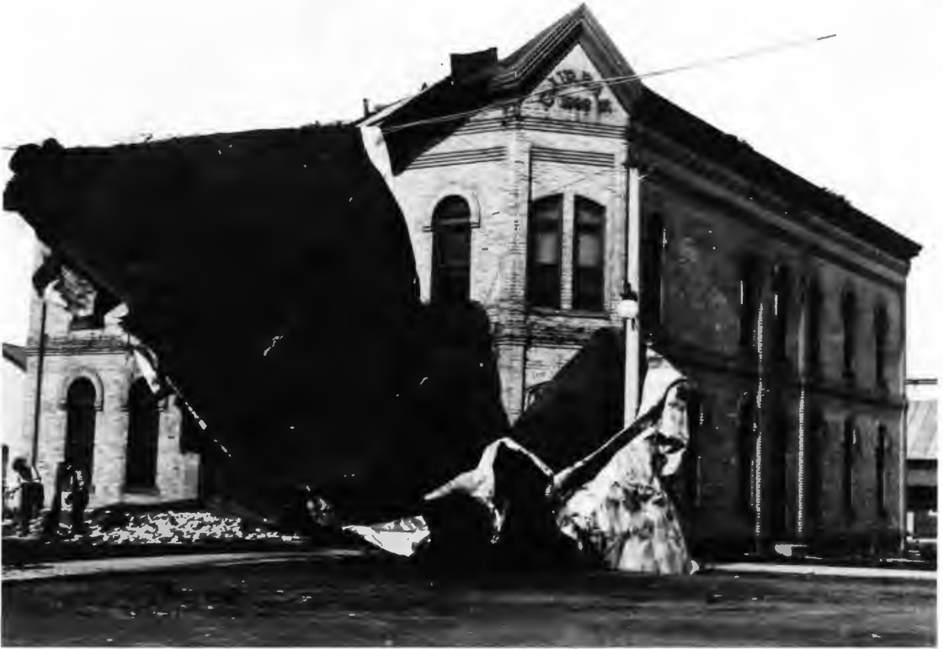
The Urban Hotel, at the Southwest corner of Ash and Water Streets, after high winds in 1904
