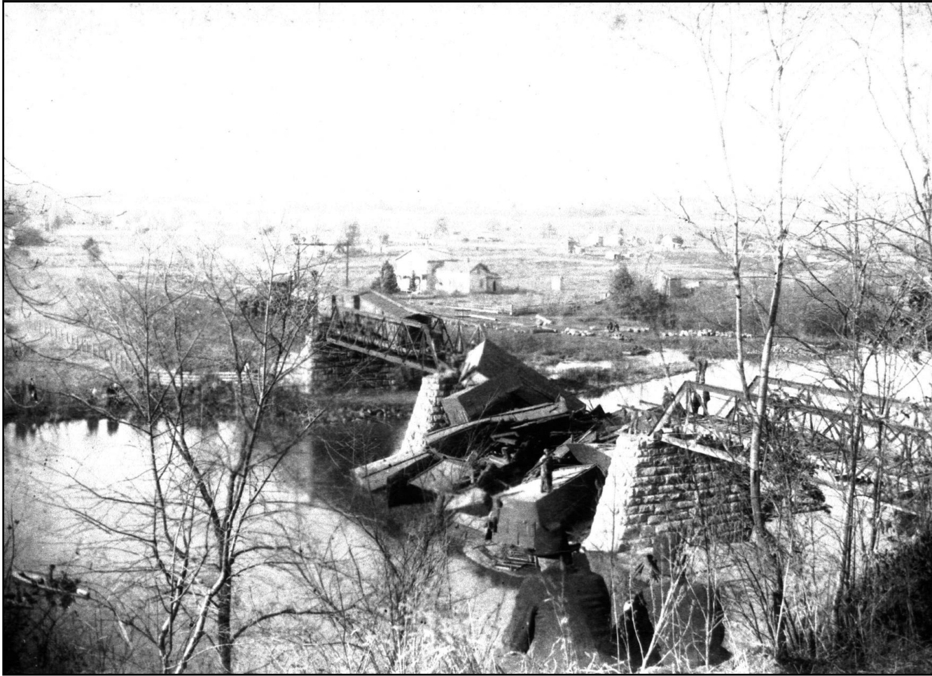
Train and bridge wreckage, circa 1890, West Baraboo, then known as Lyons
