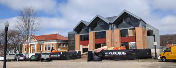
View of the whole building
