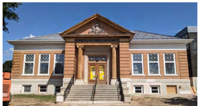
Exterior of building, old paint and roof tiles removed
