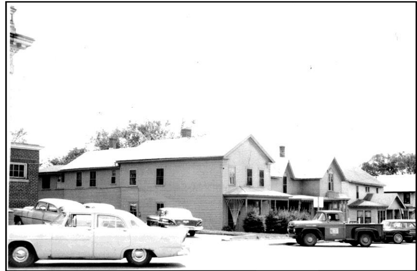
South side of 100 block of Second Avenue prior to the drive up bank
