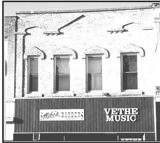
116 Third Street facade
