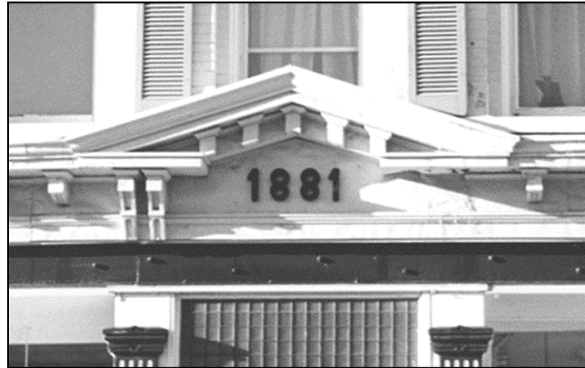
104 Third Street facade
