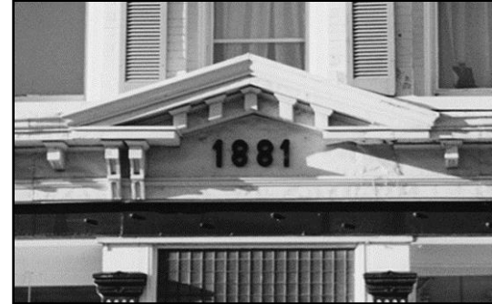
106 Third Street facade
