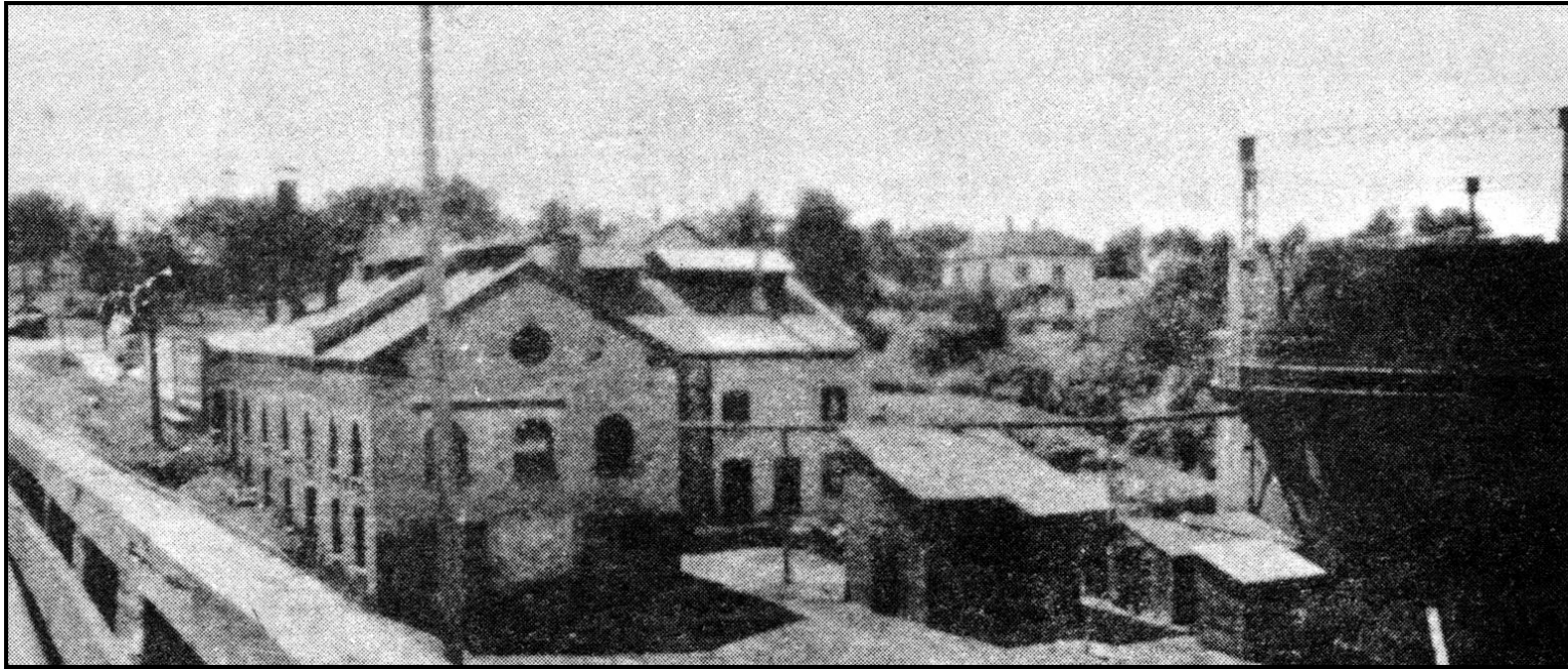
The above picture of the Baraboo Gas Holder and Plant (known as the Deep-Freeze) was featured on the July 1926 cover of the "Power and Light Company News". Picture taken from Oak Street Bridge.
